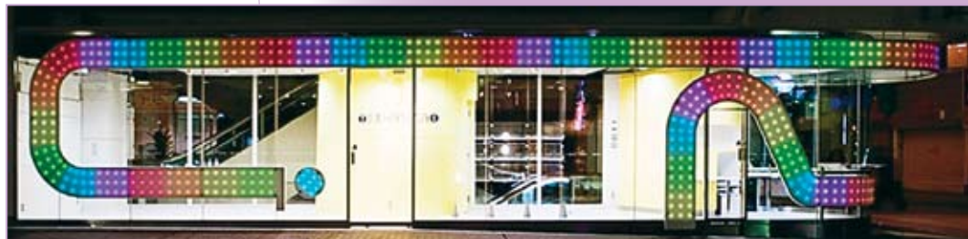
This application is one example of how Trillium color can be controlled. Each "block" of color is assigned to a different channel of a DMX control system.
